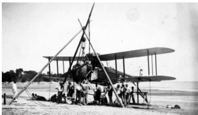
The DH.50 being refitted with wheeled undercarriage at Mindi faced a grave problem.
