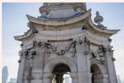
Steel cables currently hold the steeple together
